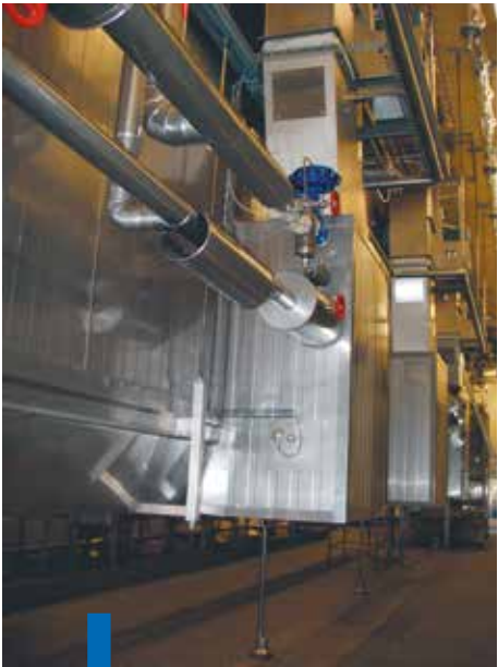
Equipment is suspended in order to achieve high hygiene standards
